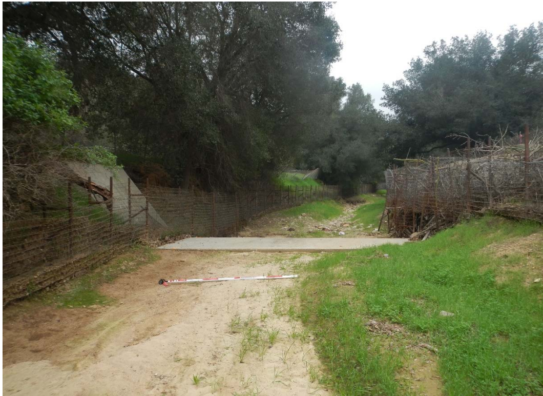
HEC-RAS RIVER STATION 12+33, DOWNSTREAM DIRECTION
