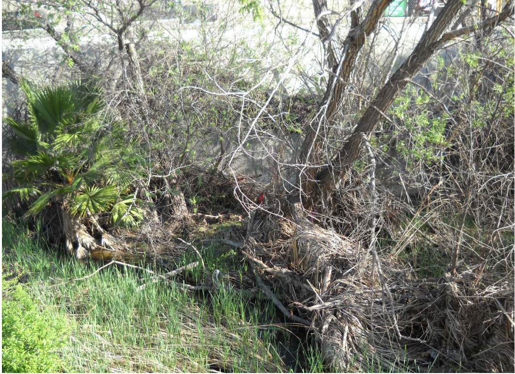
HEC-RAS RIVER STATION 60+42, CHANNEL AND LEFT BANK
