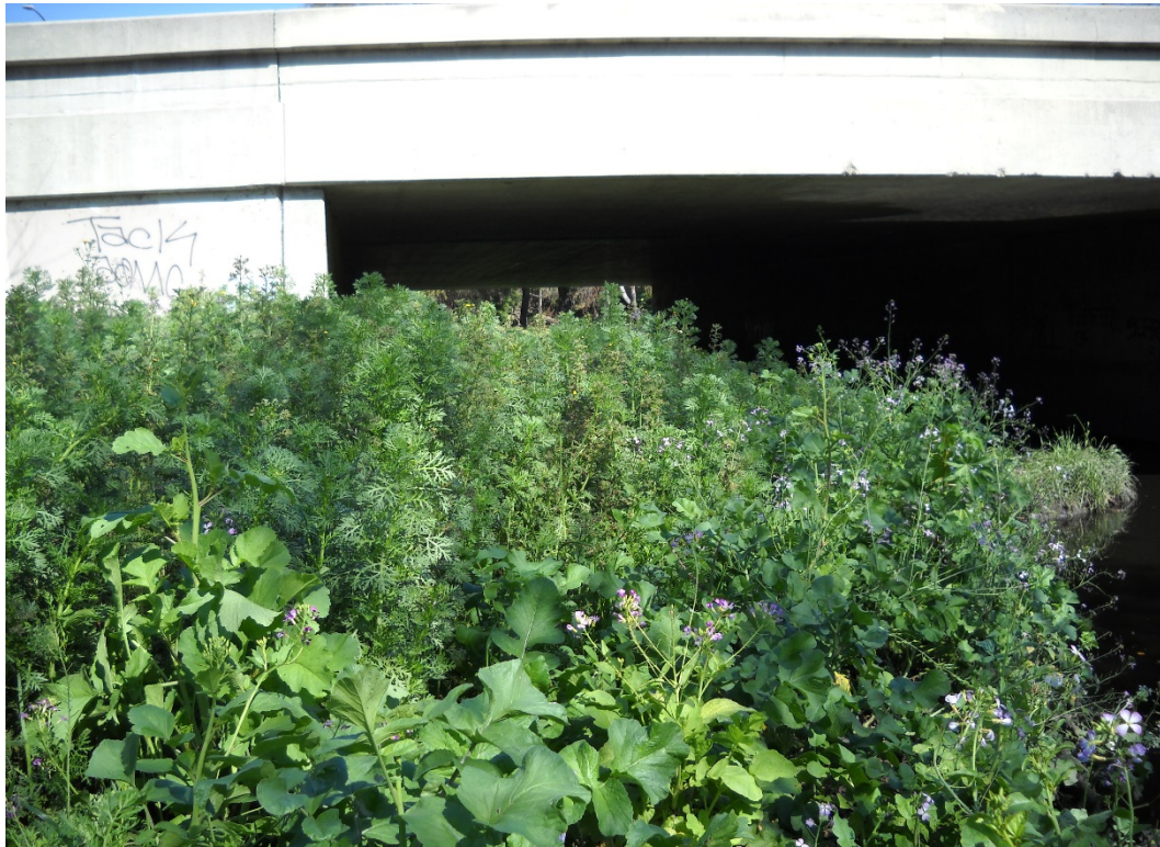
HEC-RAS RIVER STATION 5+30, UPSTREAM DIRECTION
