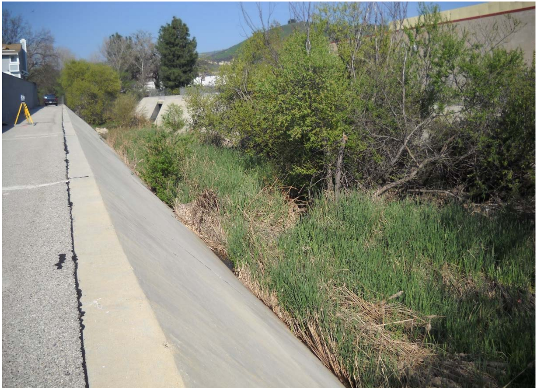
HEC-RAS RIVER STATION 60+42, UPSTREAM DIRECTION
