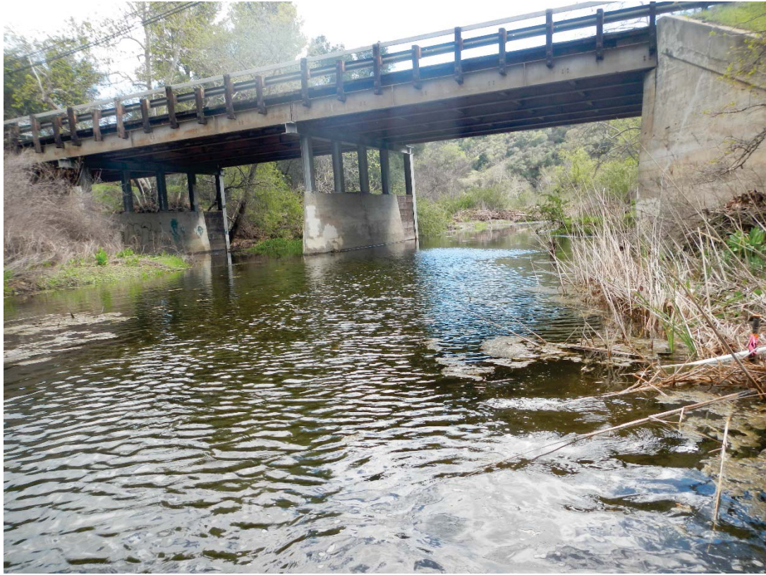
Figure 3-2. Mulholland Highway Bridge
