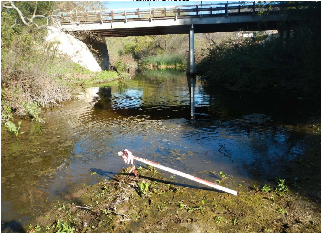
HEC-RAS RIVER STATION 10+41, UPSTREAM DIRECTION
