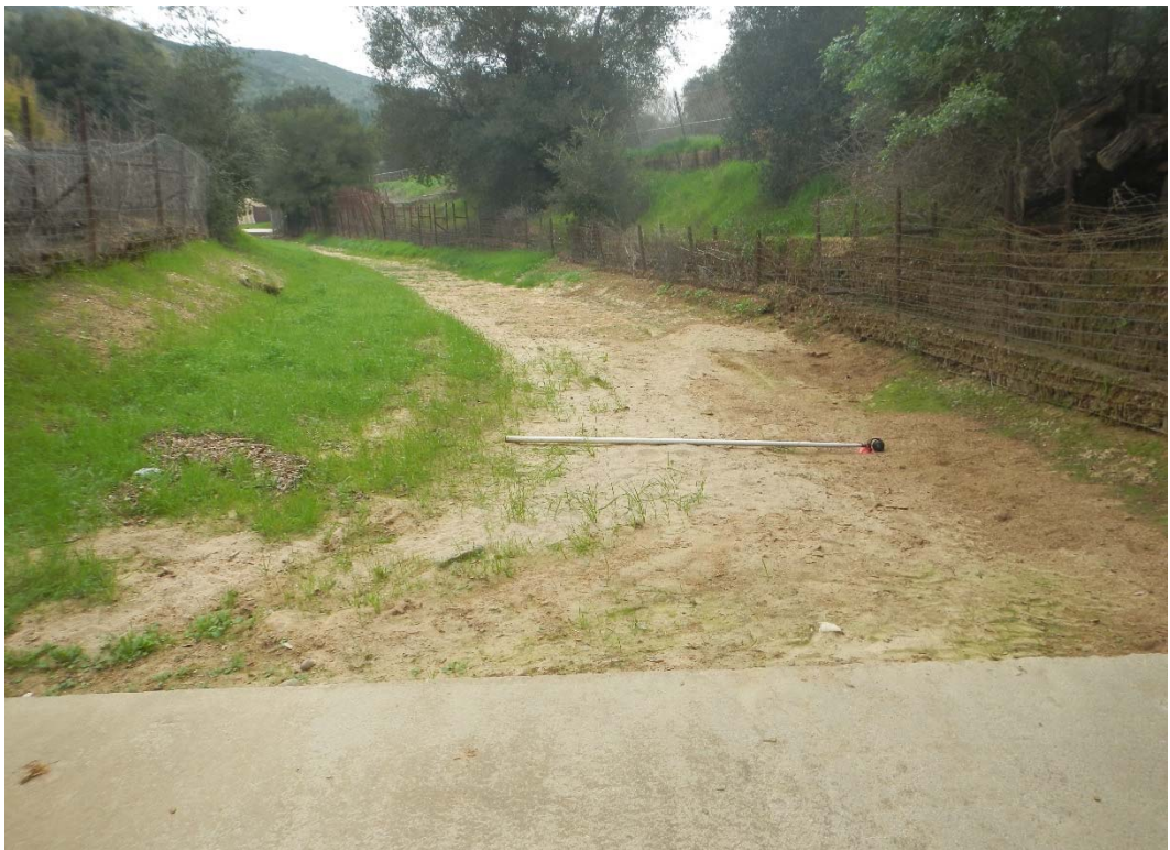
HEC-RAS RIVER STATION 12+21, UPSTREAM DIRECTION
