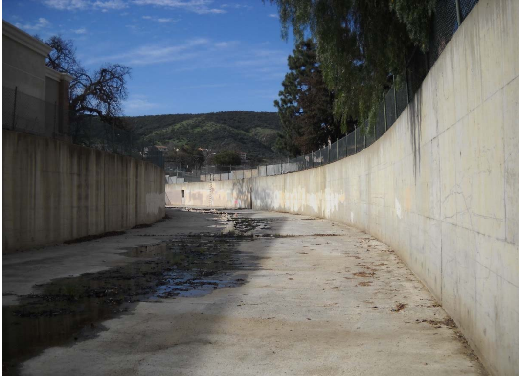
5 FT. DOWNSTREAM OF HEC-RAS RIVER STATION 4+42, DOWNSTREAM DIRECTION
