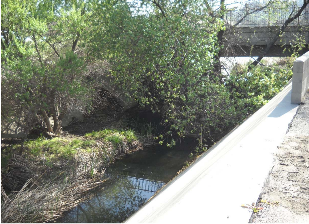
HEC-RAS RIVER STATION 60+42, DOWNSTREAM DIRECTION (THOUSAND OAKS BLVD. BRIDGE)
