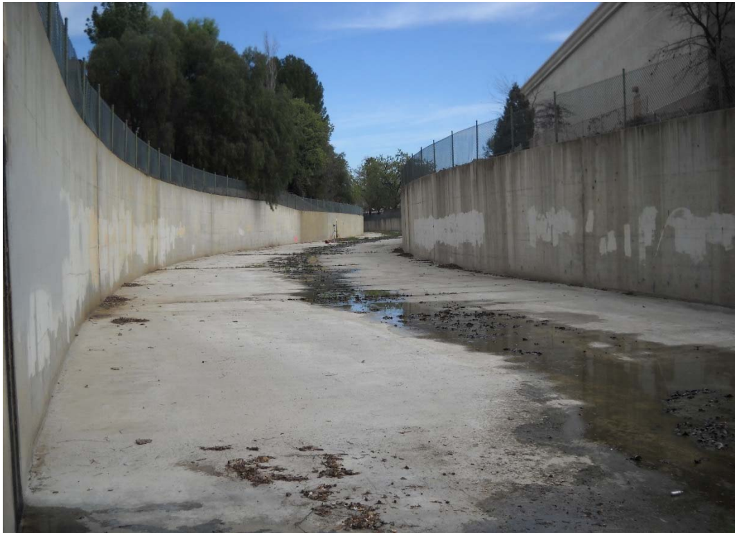
HEC-RAS RIVER STATION 00+16, UPSTREAM DIRECTION
