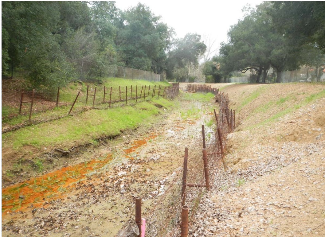
HEC-RAS RIVER STATION 29+52, DOWNSTREAM DIRECTION
