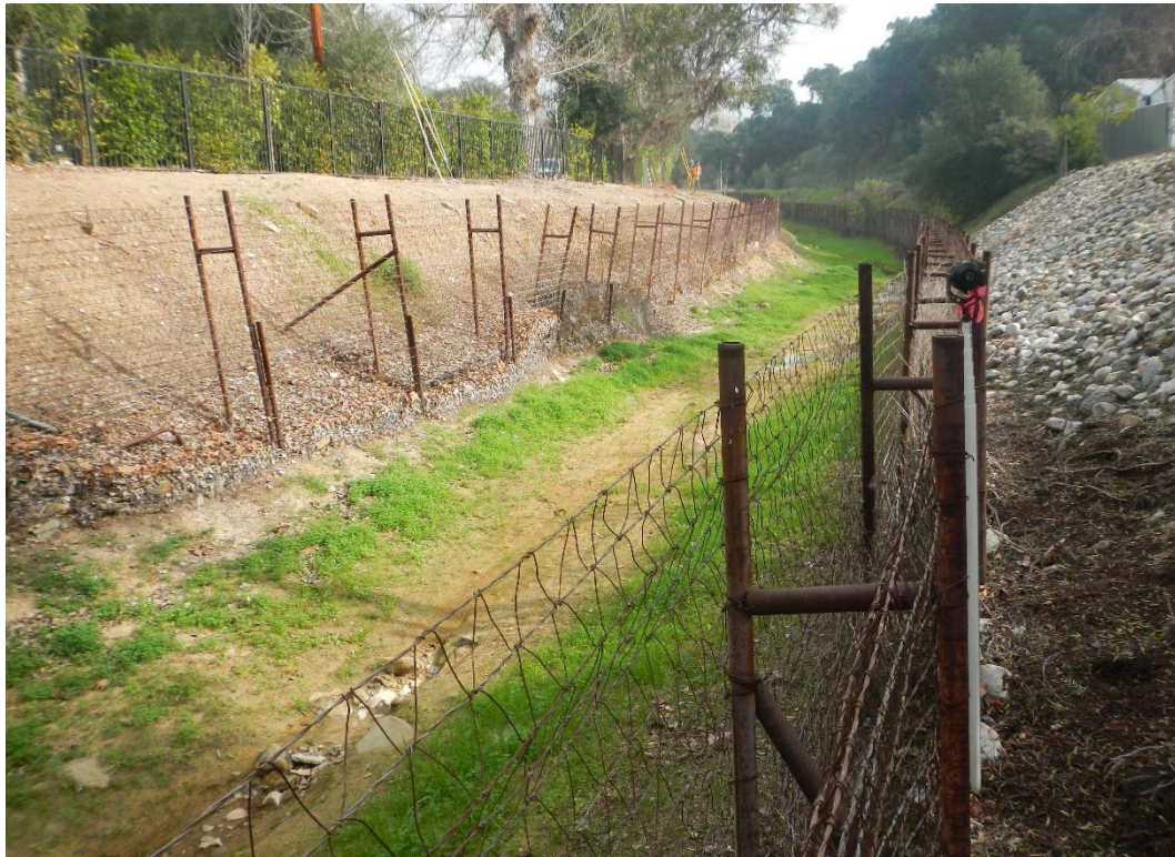
HEC-RAS RIVER STATION 21+54, UPSTREAM DIRECTION
