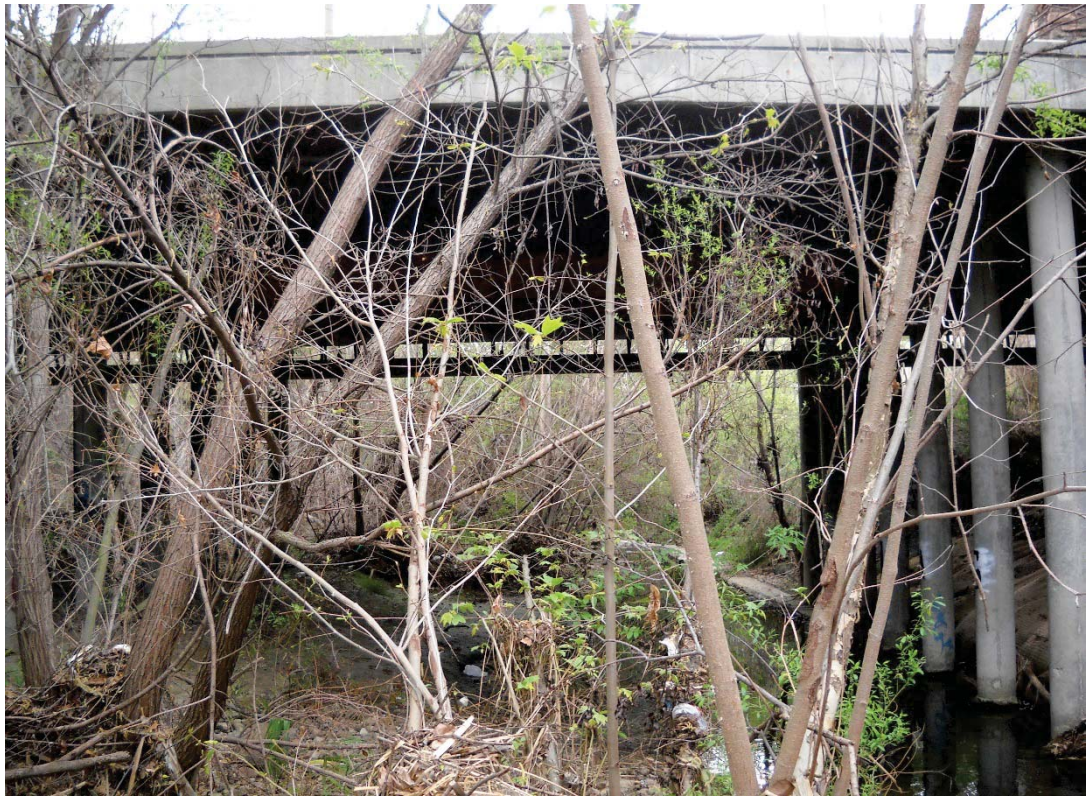
Figure 6-5. Oak Creek Lane Bridge
