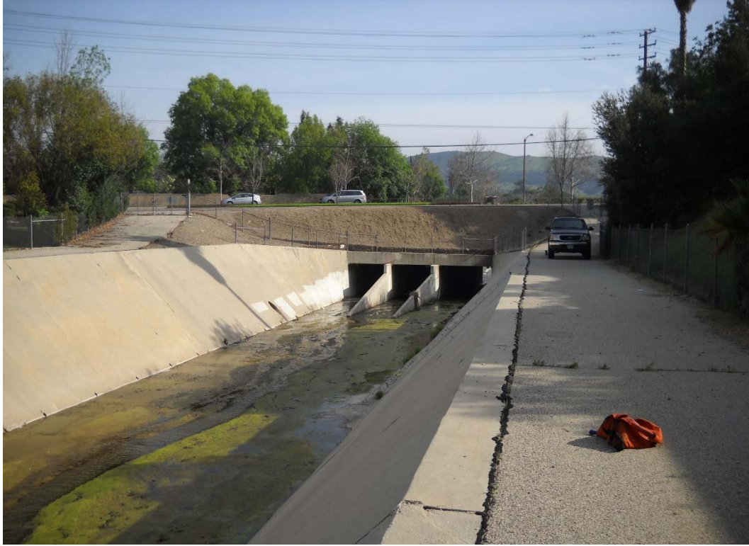
22 FT. DOWNSTREAM OF HEC-RAS RIVER STATION 48+22, DOWNSTREAM DIRECTION (KANAN RD. CULVERT)
