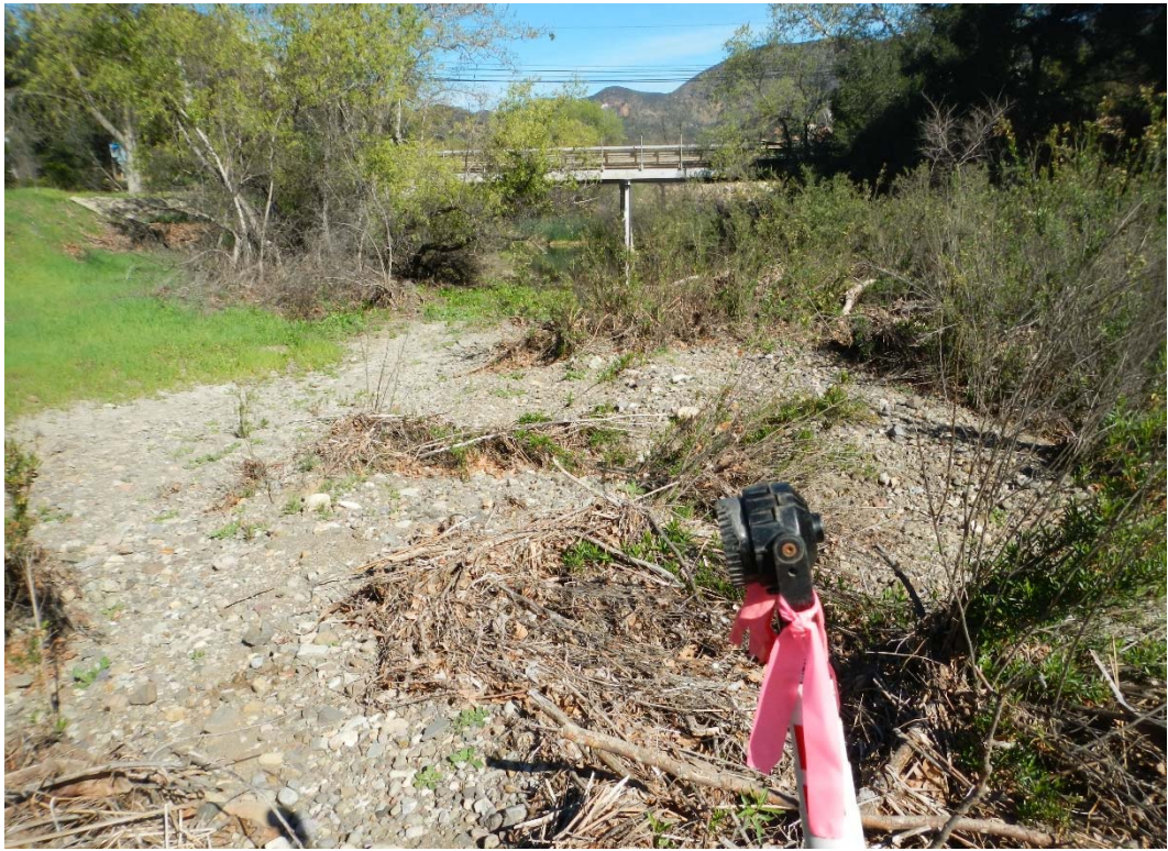
HEC-RAS RIVER STATION 9+21, UPSTREAM DIRECTION
