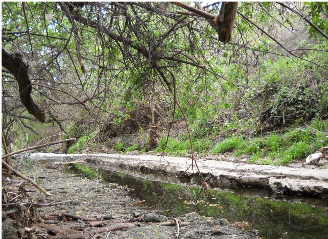
HEC-RAS RIVER STATION 31+89, DOWNSTREAM DIRECTION
