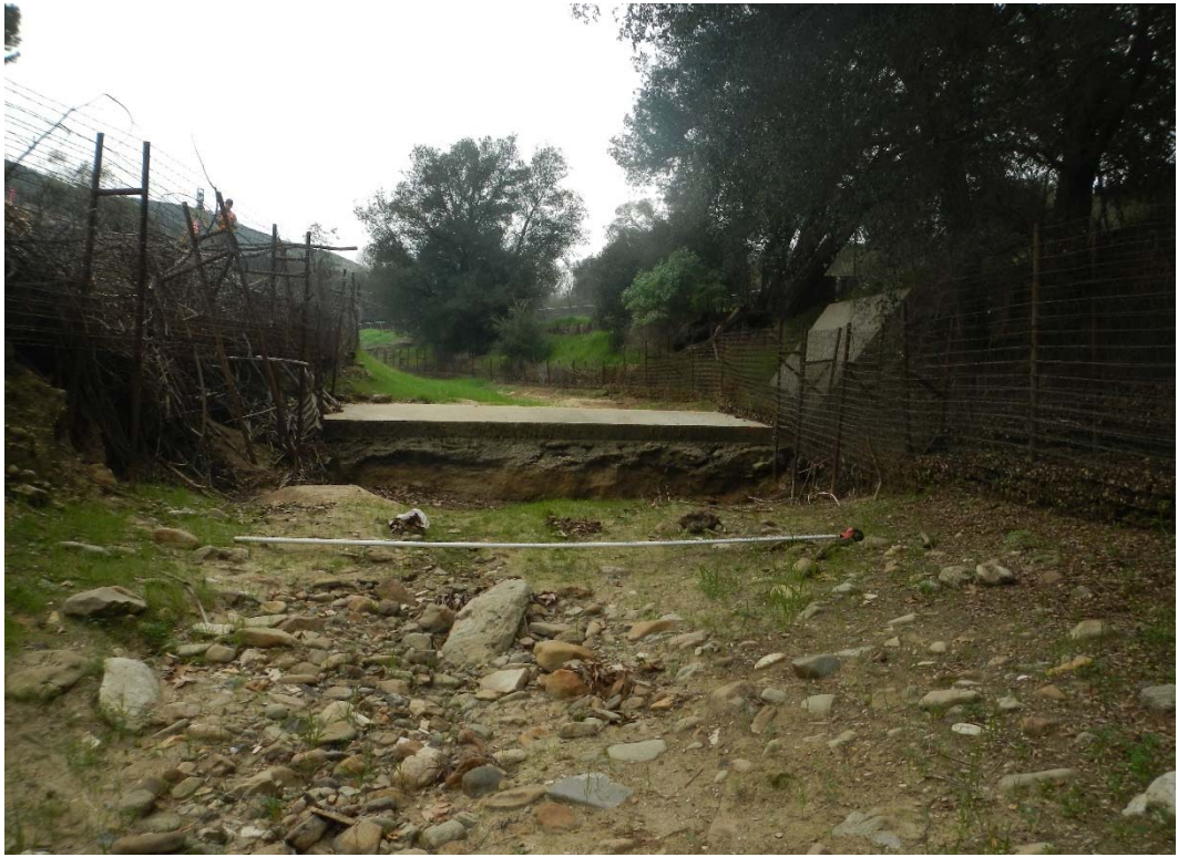
HEC-RAS RIVER STATION 11+78, UPSTREAM DIRECTION
