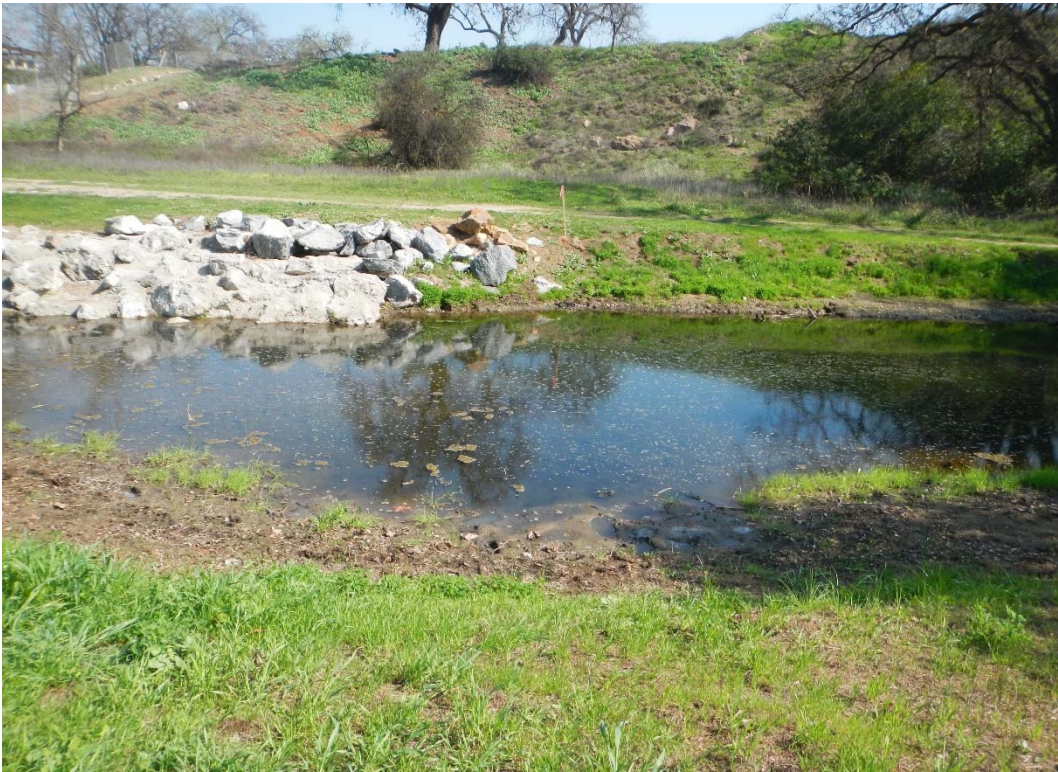
REACH UPSTREAM EXTENT, HEC-RAS RIVER STATION 11+15, CHANNEL
