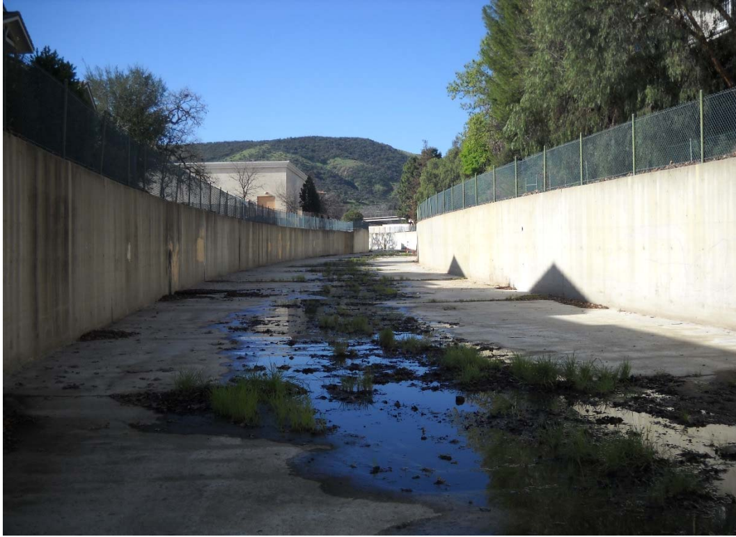
HEC-RAS RIVER STATION 7+00, DOWNSTREAM DIRECTION
