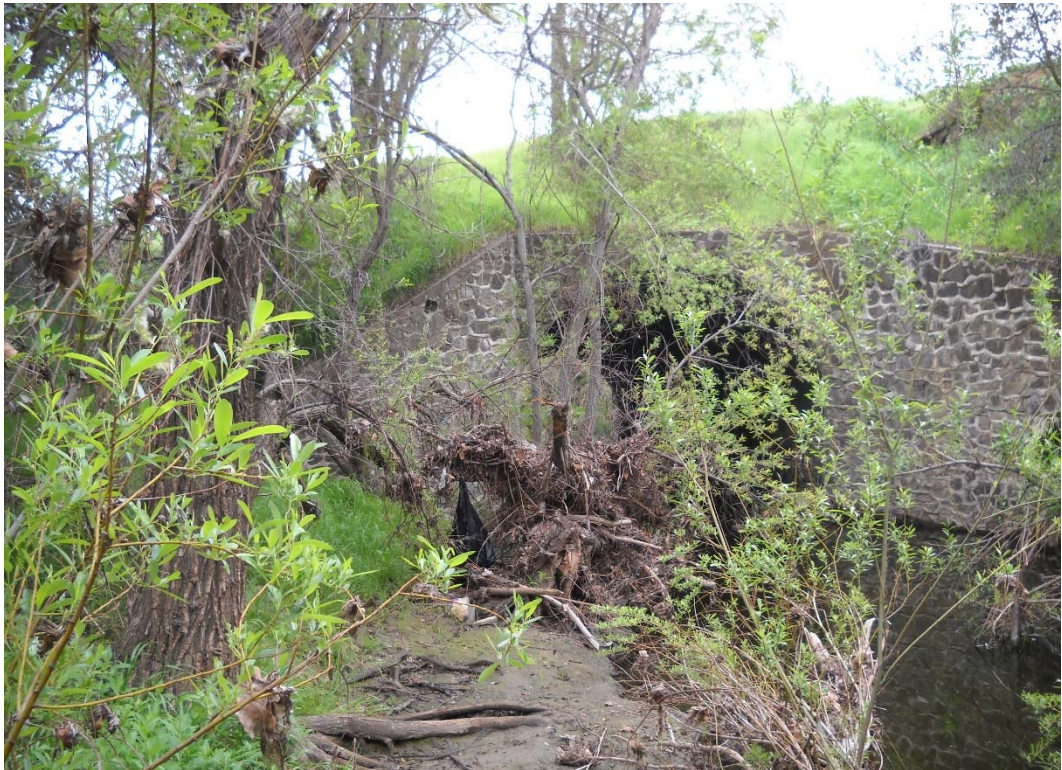
HEC-RAS RIVER STATION 0+78, DOWNSTREAM DIRECTION
