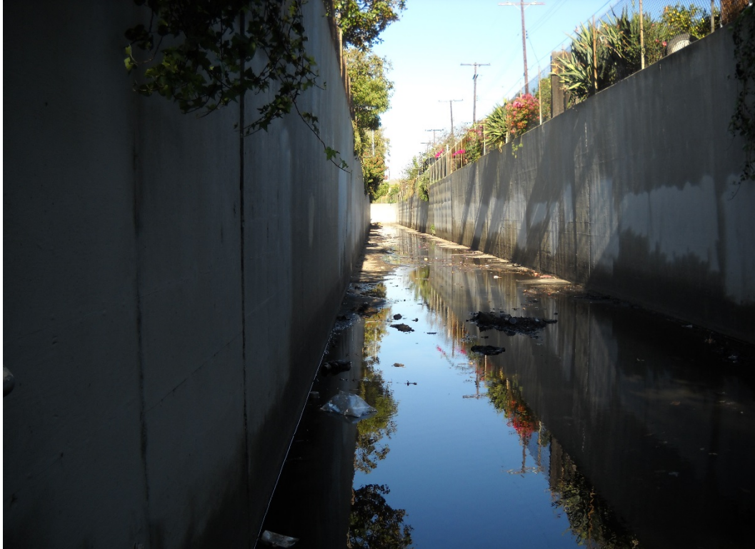
REACH UPSTREAM EXTENT, HEC-RAS RIVER STATION 12+06, UPSTREAM DIRECTION
