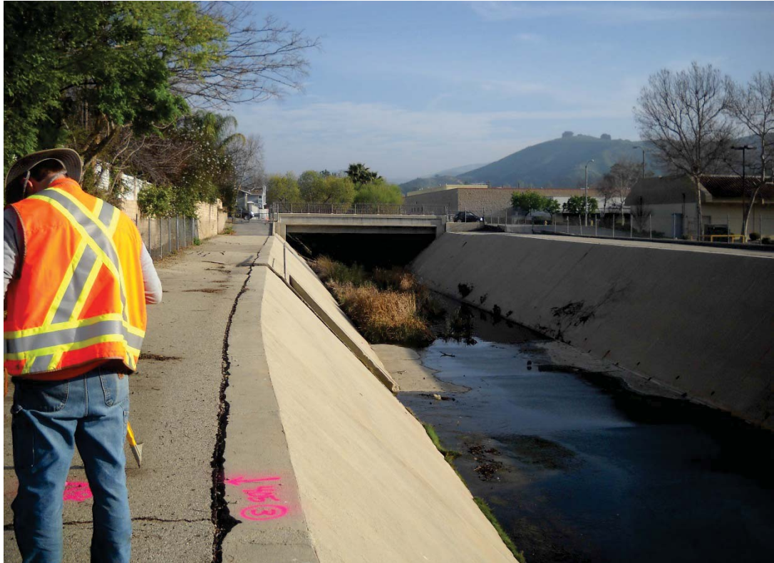
Figure 6-2. E. Thousand Oaks Blvd. Bridge
