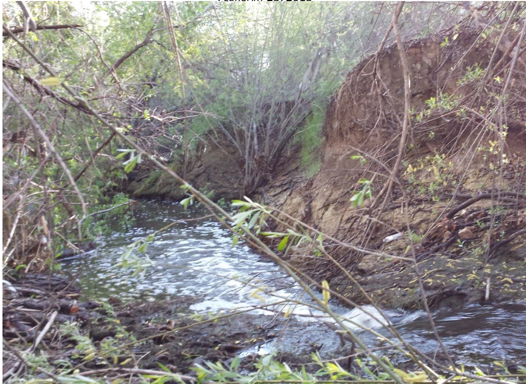
HEC-RAS RIVER STATION 29+58, DOWNSTREAM DIRECTION
