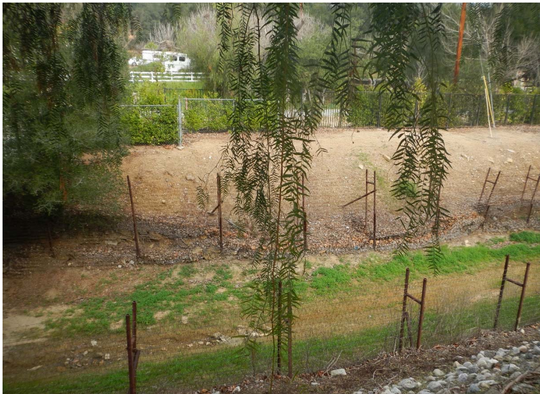
HEC-RAS RIVER STATION 21+54, CHANNEL & RIGHT BANK
