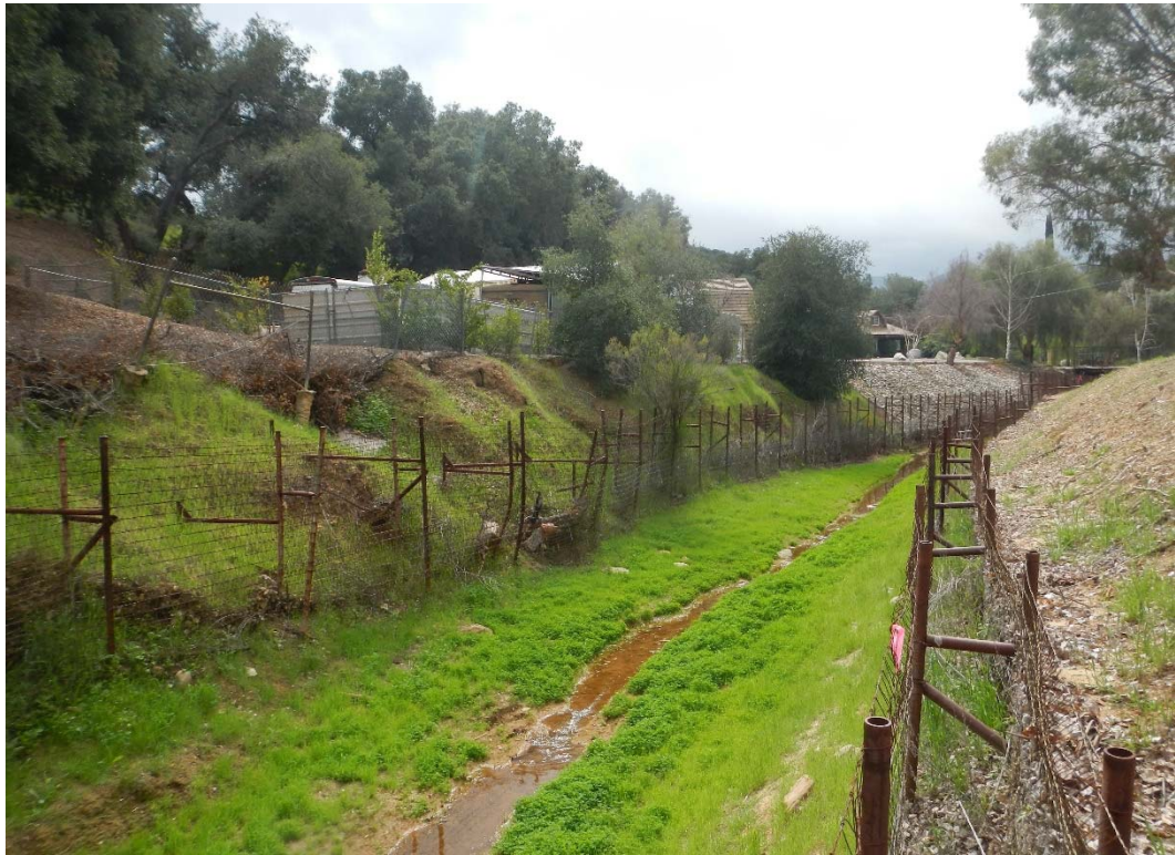
HEC-RAS RIVER STATION 24+32, DOWNSTREAM DIRECTION
