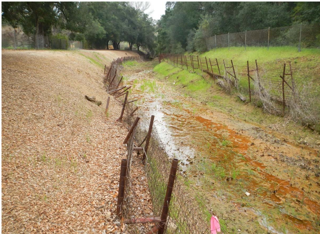
HEC-RAS RIVER STATION 26+96, UPSTREAM DIRECTION
