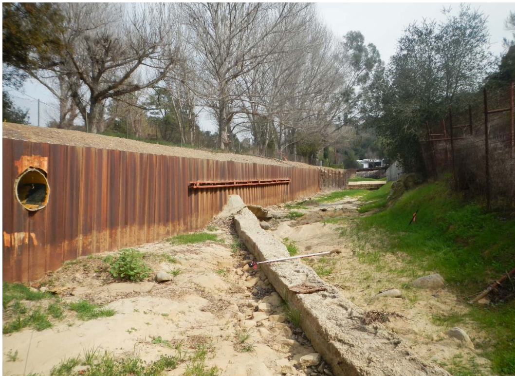
HEC-RAS RIVER STATION 17+54, UPSTREAM DIRECTION
