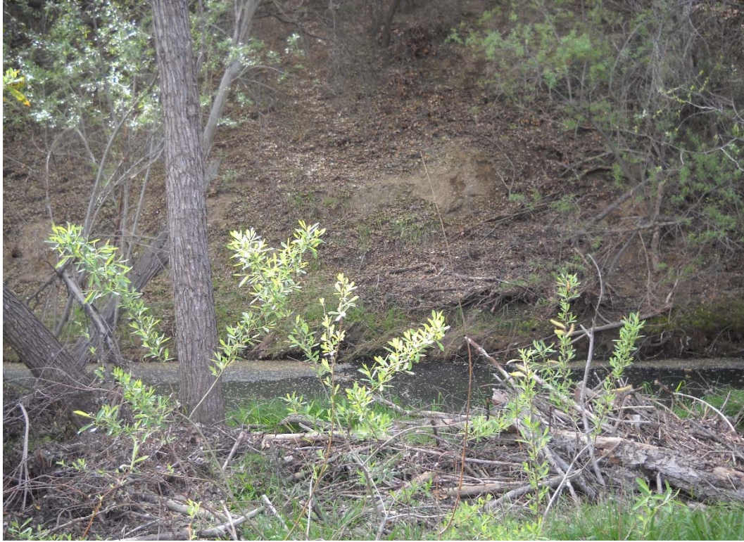
HEC-RAS RIVER STATION 72+57, CHANNEL AND RIGHT BANK
