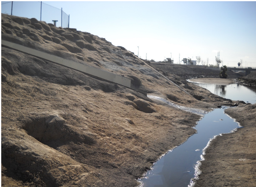
HEC-RAS RIVER STATION 01+01, DOWNSTREAM DIRECTION
