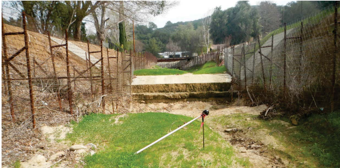
Figure 5-3. Stokes Canyon Channel Concrete Section (1 of 3 Structures)
