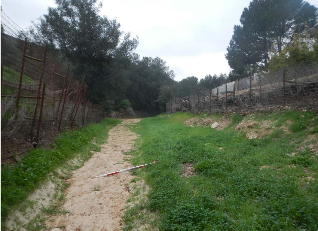
HEC-RAS RIVER STATION 13+95, DOWNSTREAM DIRECTION
