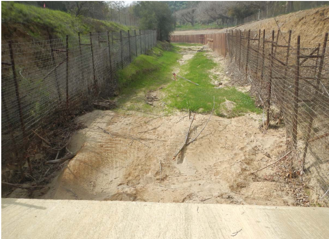
11FT. DOWNSTREAM OF HEC-RAS RIVER STATION 19+54, DOWNSTREAM DIRECTION
