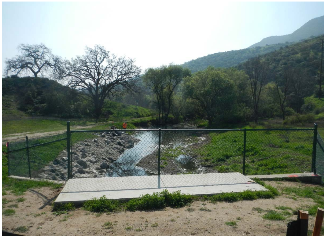
HEC-RAS RIVER STATION 12+00, DOWNSTREAM DIRECTION
