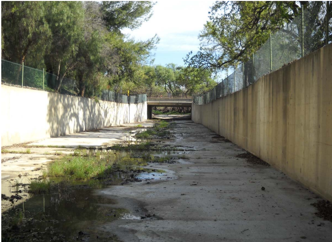
HEC-RAS RIVER STATION 7+00, UPSTREAM DIRECTION (DRIVER AVE. BRIDGE)
