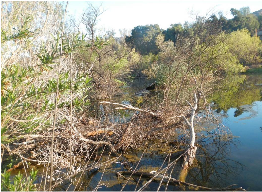
49 FT. UPSTREAM OF HEC-RAS RIVER STATION 4+51, UPSTREAM DIRECTION
