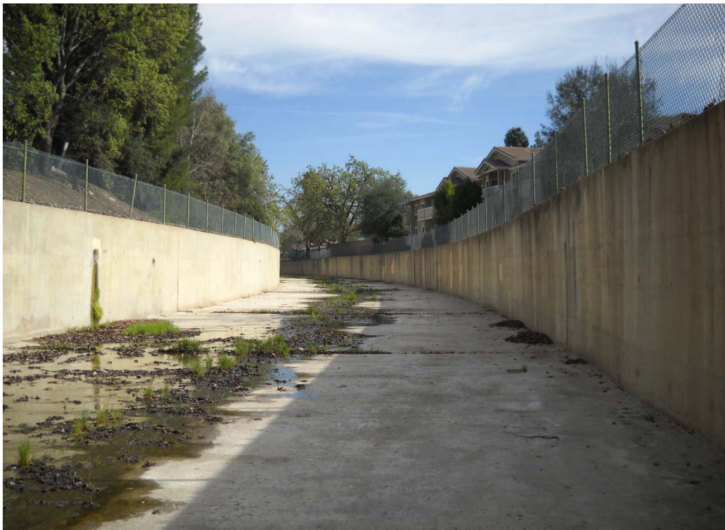
77 FT. UPSTREAM OF HEC-RAS RIVER STATION 3+40, UPSTREAM DIRECTION
