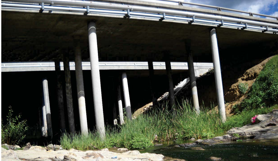
Figure 6-11. Roadside Drive Bridge
