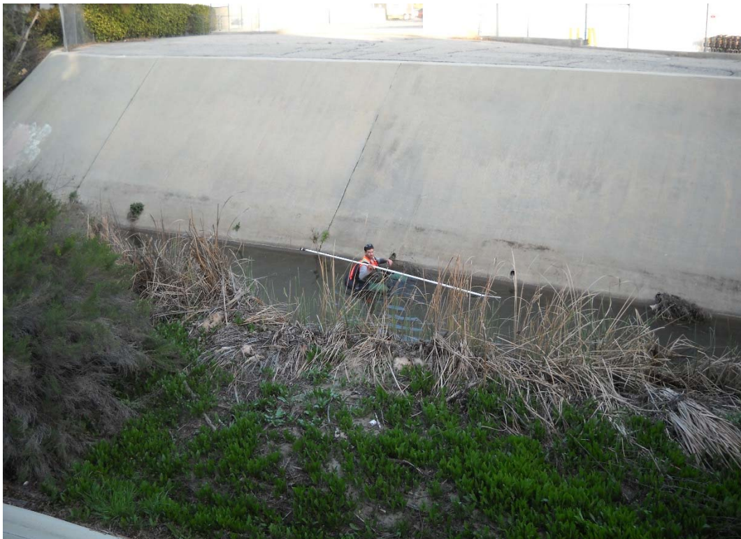
62 FT. UPSTREAM OF HEC-RAS RIVER STATION 64+38, CHANNEL AND LEFT BANK
