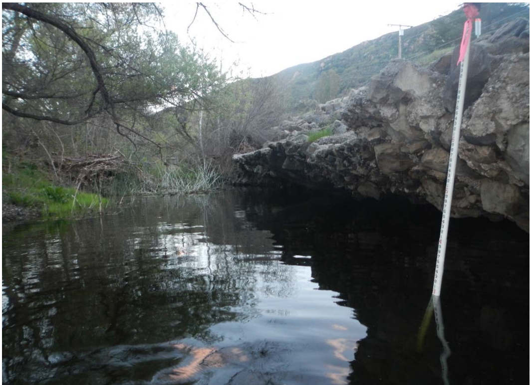
HEC-RAS RIVER STATION 15+39, DOWNSTREAM DIRECTION
