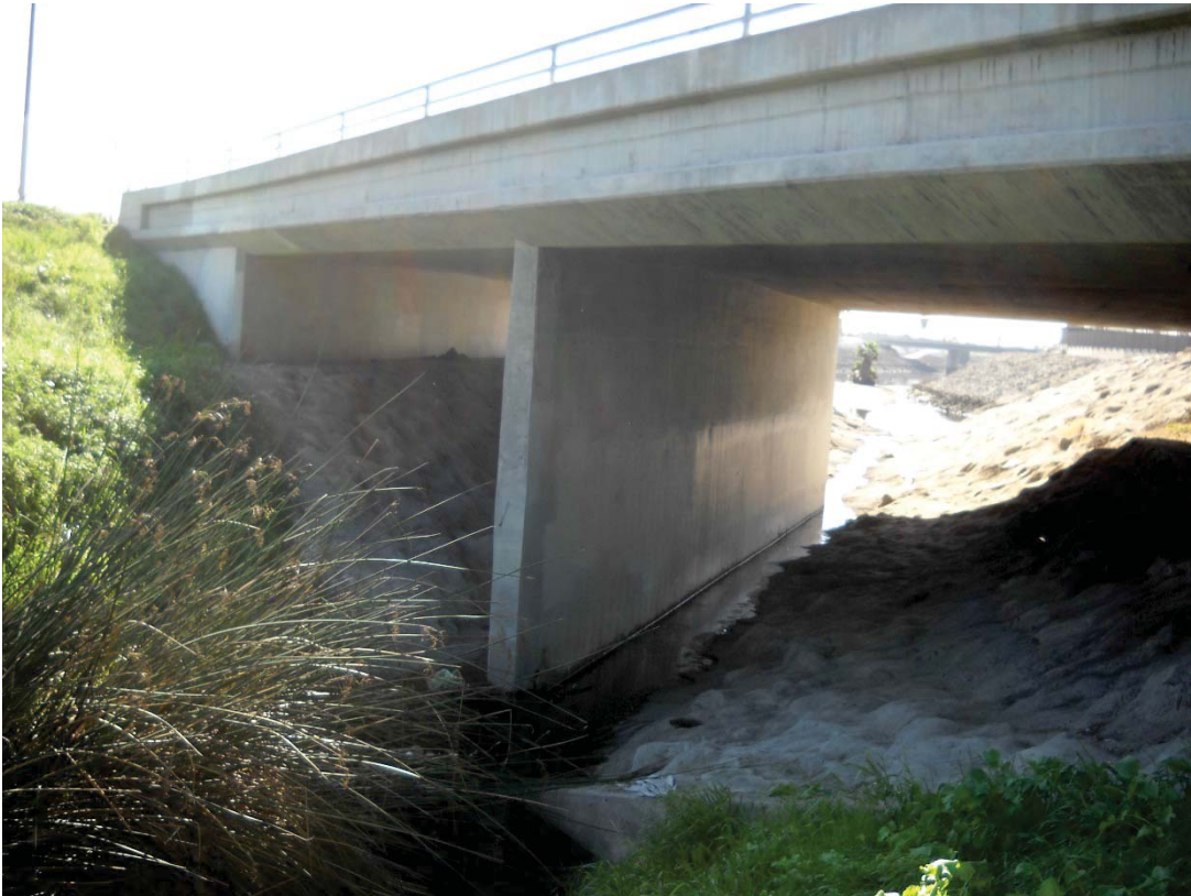
Figure 2-3. Park ‘n Ride Access Bridge
