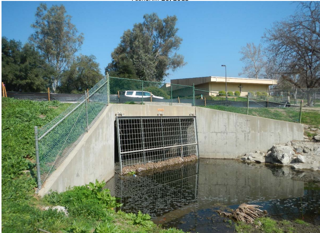
HEC-RAS RIVER STATION 12+00, UPSTREAM DIRECTION
