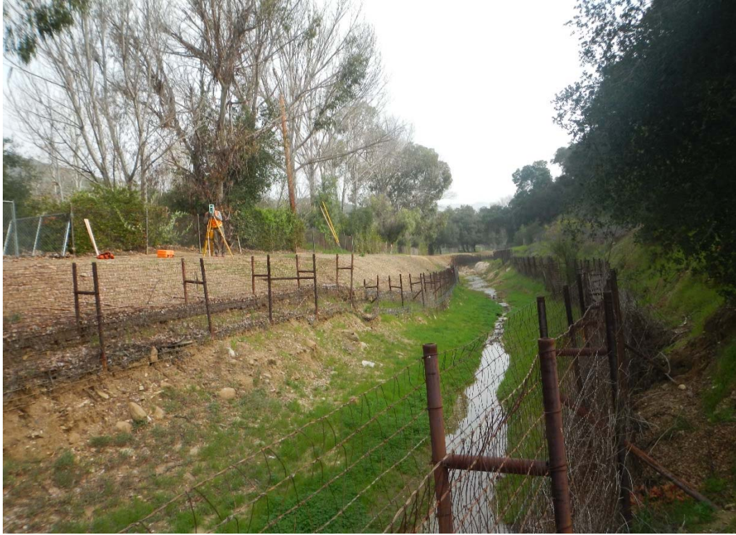
92 FT. UPSTREAM OF HEC-RAS RIVER STATION 22+78, UPSTREAM DIRECTION
