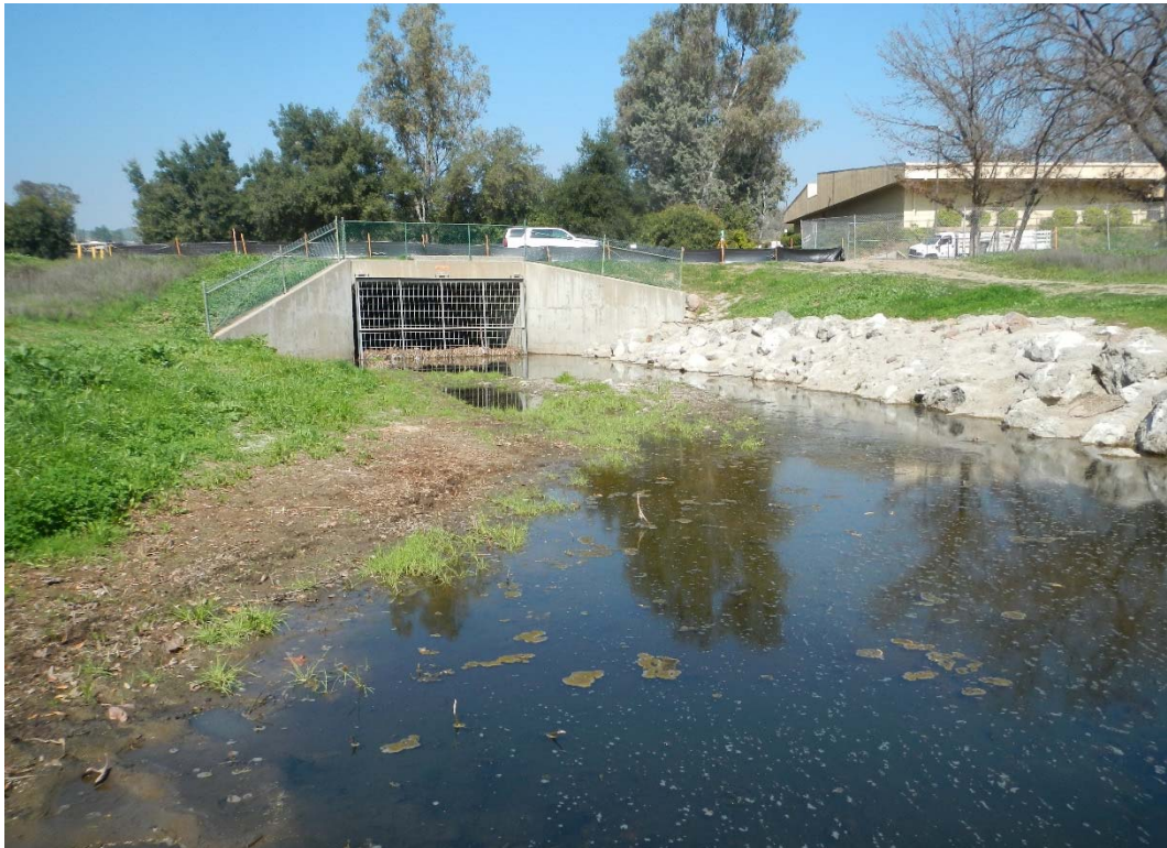
REACH UPSTREAM EXTENT, HEC-RAS RIVER STATION 11+15, UPSTREAM DIRECTION
