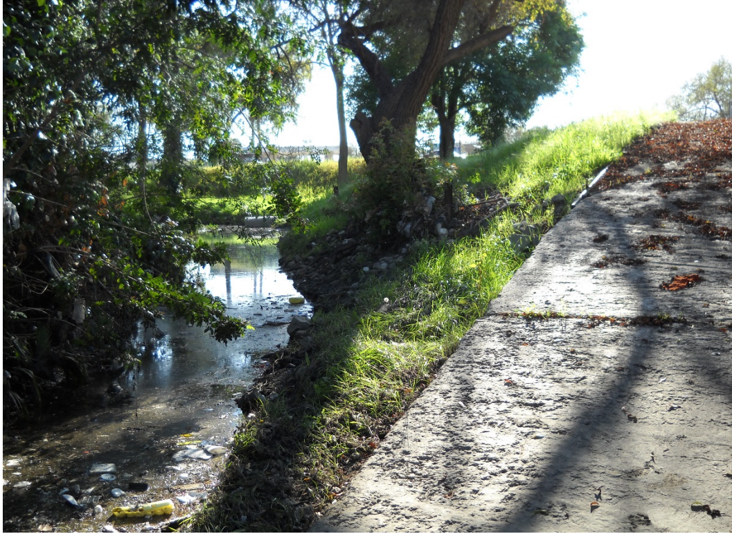
REACH UPSTREAM EXTENT, HEC-RAS RIVER STATION 12+06, DOWNSTREAM DIRECTION
