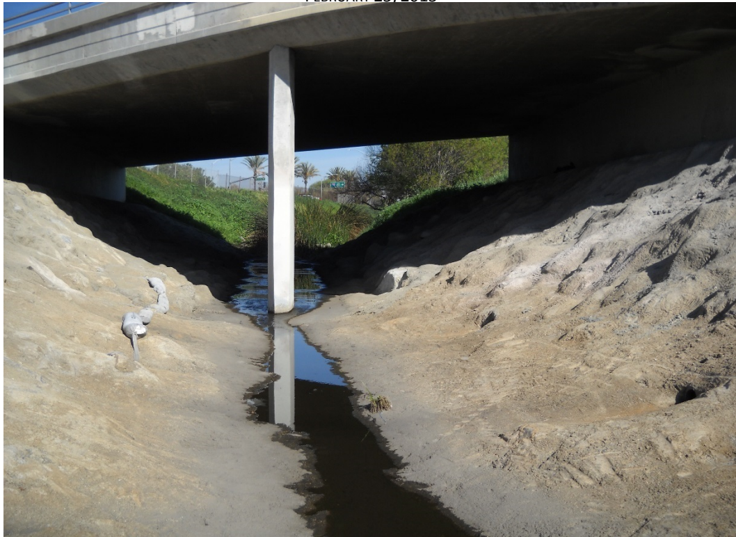
HEC-RAS RIVER STATION 01+01, UPSTREAM DIRECTION
