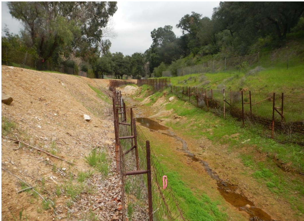
HEC-RAS RIVER STATION 24+32, UPSTREAM DIRECTION
