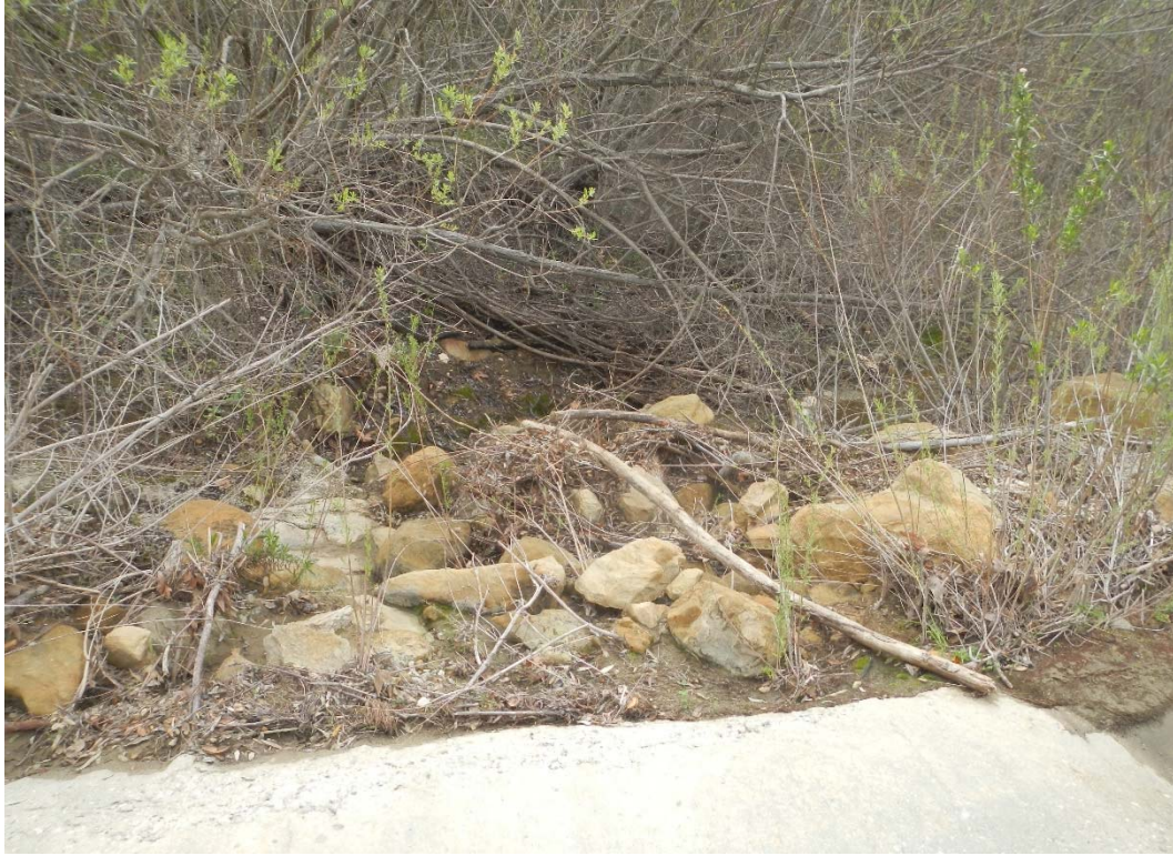
HEC-RAS RIVER STATION 33+47, DOWNSTREAM DIRECTION
