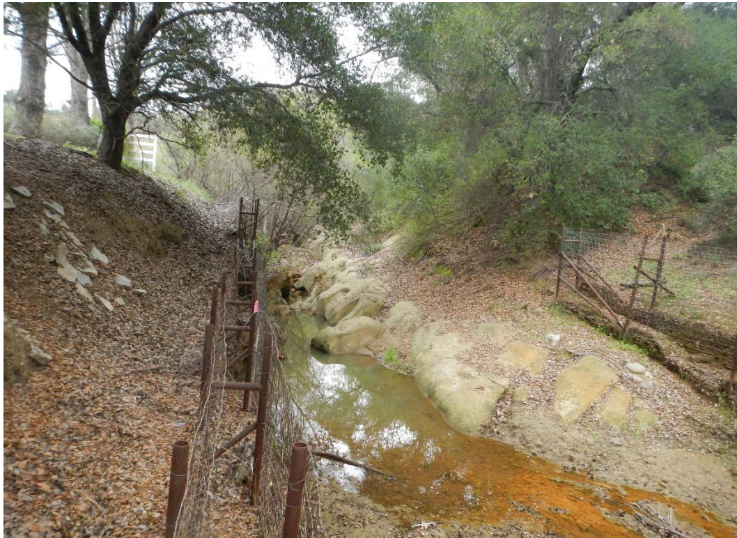
REACH UPSTREAM EXTENT, HEC-RAS RIVER STATION 30+92, UPSTREAM DIRECTION
