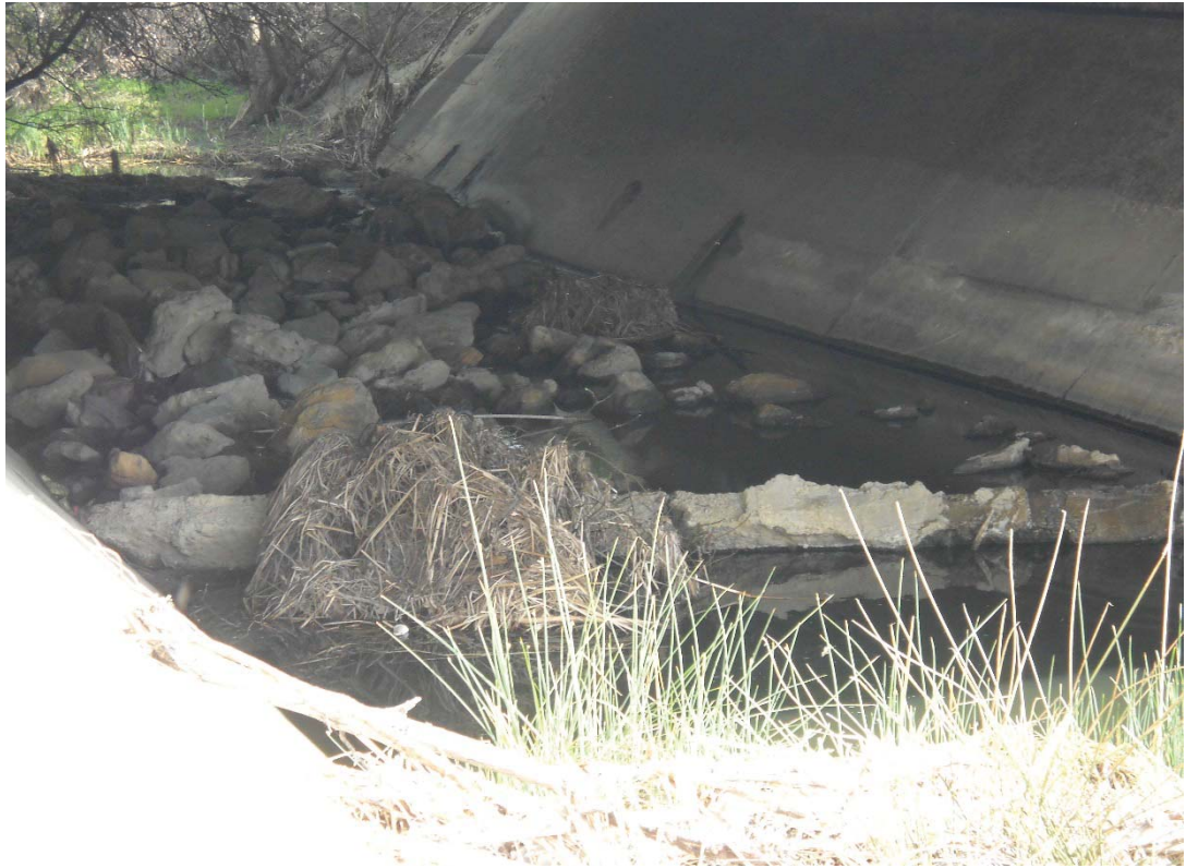
Figure 6-3. Beneath E. Thousand Oaks Blvd. Bridge
