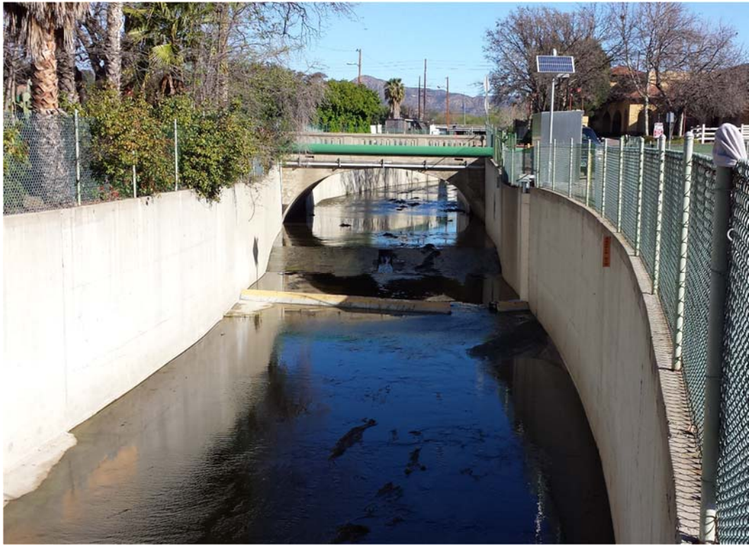
HEC-RAS RIVER STATION 14+25, UPSTREAM DIRECTION (AGOURA RD. BRIDGE)
