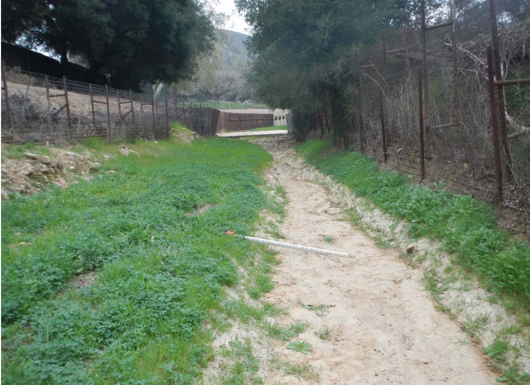
HEC-RAS RIVER STATION 13+95, UPSTREAM DIRECTION
