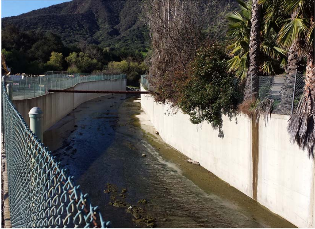
HEC-RAS RIVER STATION 14+25, DOWNSTREAM DIRECTION
