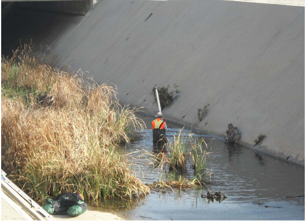
HEC-RAS RIVER STATION 57+19, UPSTREAM DIRECTION
