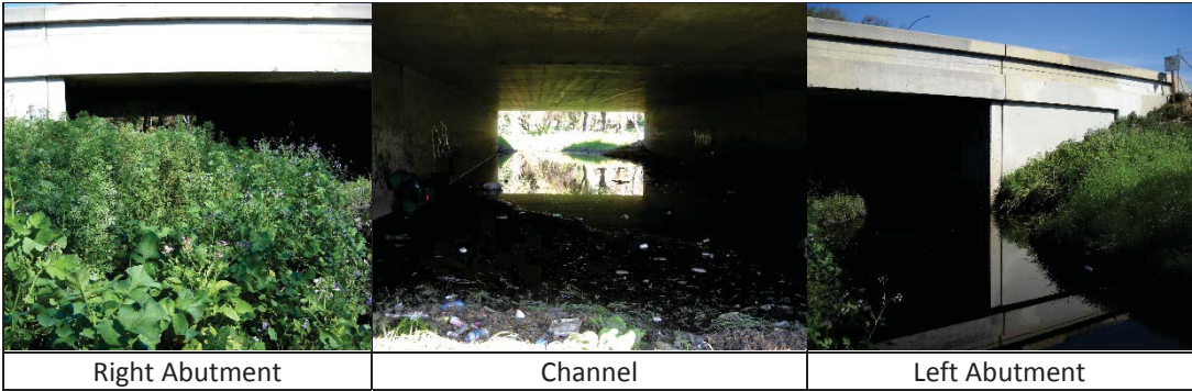
Figure 2-2. Artesia Blvd Bridge
