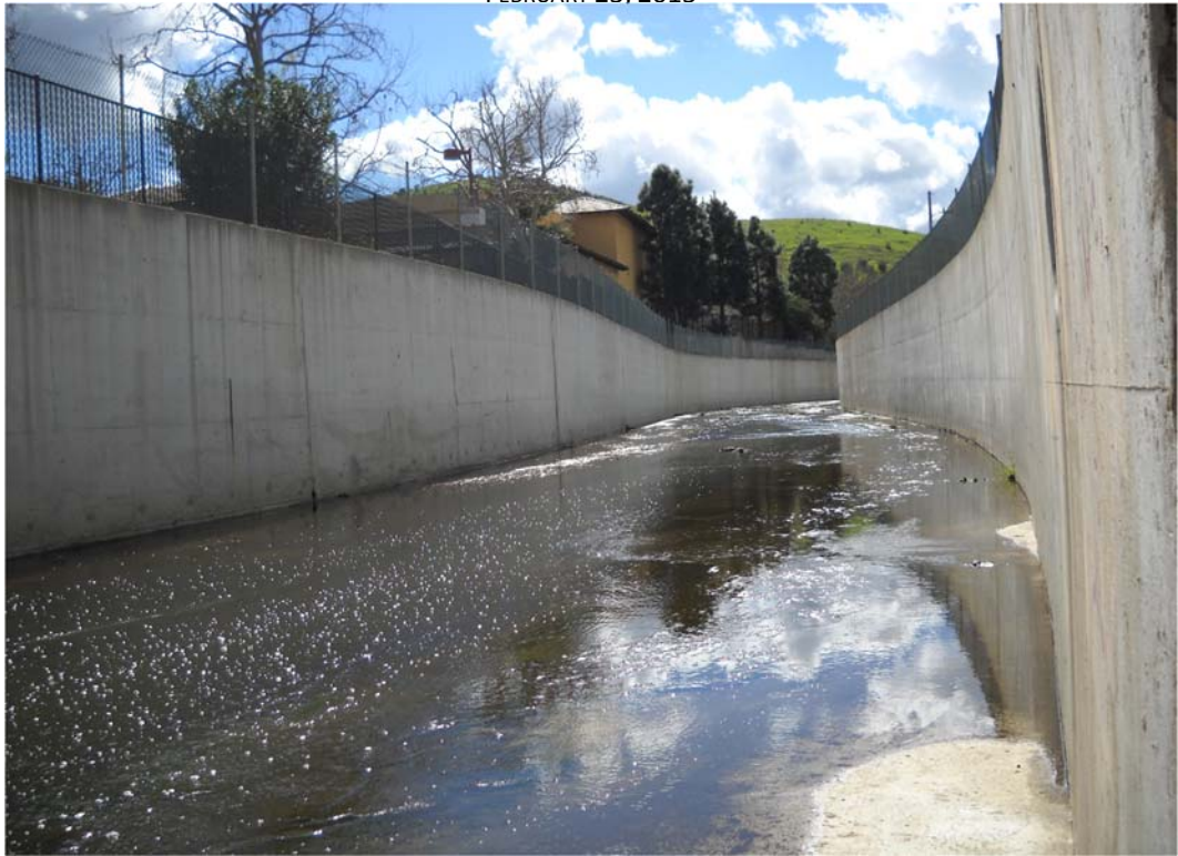
HEC-RAS RIVER STATION 22+42, DOWNSTREAM DIRECTION
